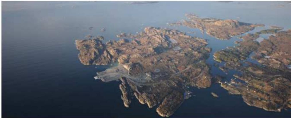
Veolia's decommissioning site in Lutelandet - Norway
