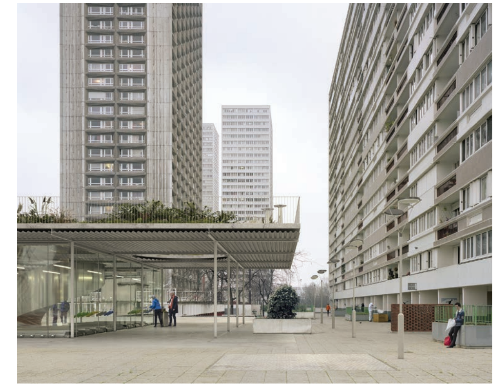
The "central waste plant" in the city
